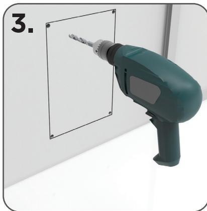
3. Drill a hole in each of the 4 inside corners with a minimum of 10mm(3/8") drill bit.
