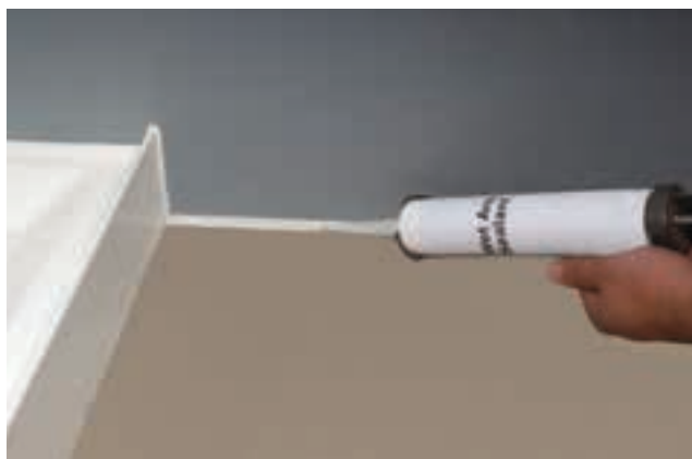
Figure 60: Seal Floor and Wall Junctions
