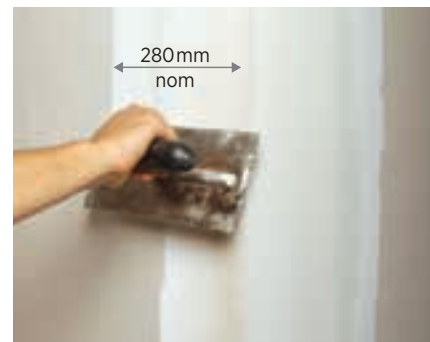
4. Apply third coat to corner faces
