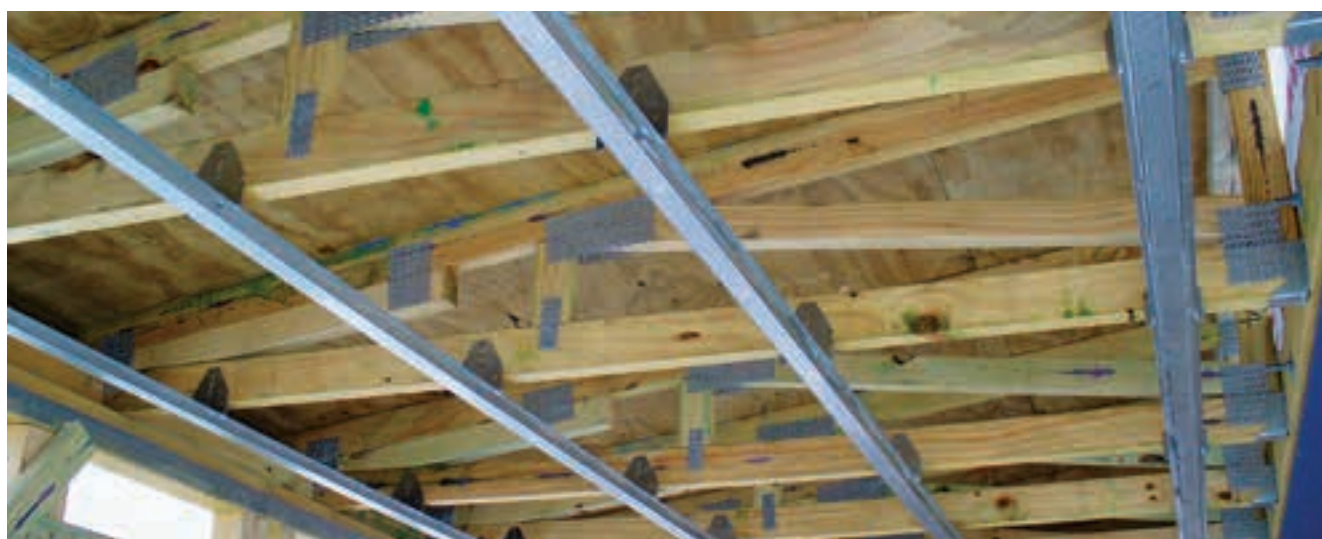
Figure 16: Furred Ceiling Direct Fixed
