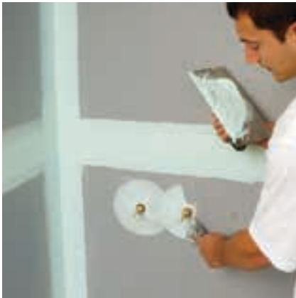
4. Apply skim coat of setting compound at joints and around penetrations.
