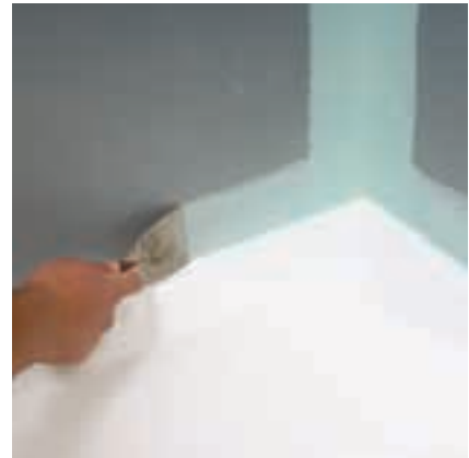
6. Apply skim coat of setting compound at sheet base.
