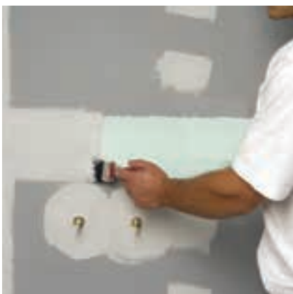
7. Apply two liberal coats of wet area seal coat at all joints, junctions, penetrations and fastener heads.
