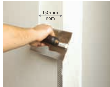
2. Apply first coat to both corner faces
