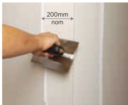
3. Apply second coat to corner faces
