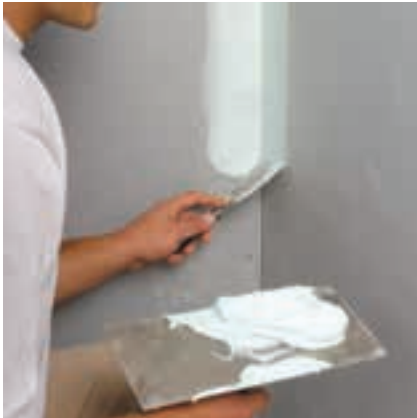
1. Apply bedding coat of USG Boral setting compound.
