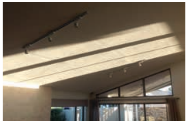
Figure 6: Same plasterboard surface under glancing light
