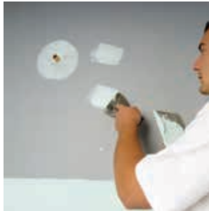
5. Apply skim coat of setting compound to fastener heads.
