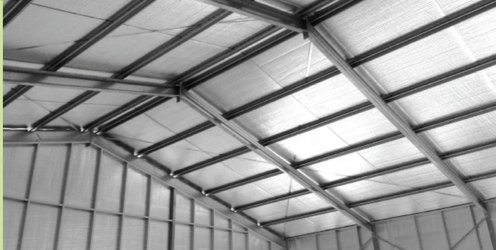
ThermalLiner™ is an Extra Heavy Duty three-in-one reflective insulation, thermal break and Class 2 Vapour Barrier. ThermalLiner™ is suitable for use in roof, wall and floor applications. Designed to manage heat gain and heat loss, ThermalLiner™ offers superior thermal performance to conventional insulation, and reduces thermal bridging and conductivity between building elements.
