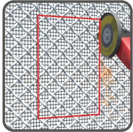
Take the measurements needed to cut the opening by following Steps 1-3 of the previous instructions. Using an angle grinder, cut out the opening.
