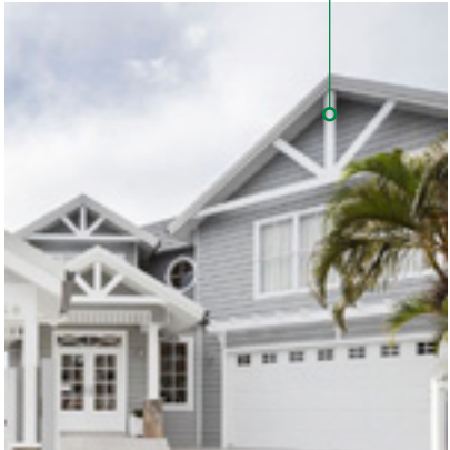
Open gable with King Post trusses
