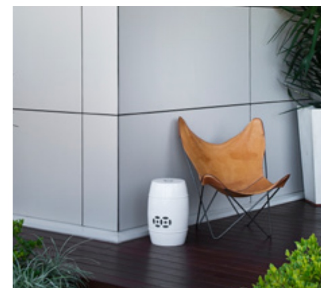
Matrix™ Cladding Horizontal layout with joints painted black.
