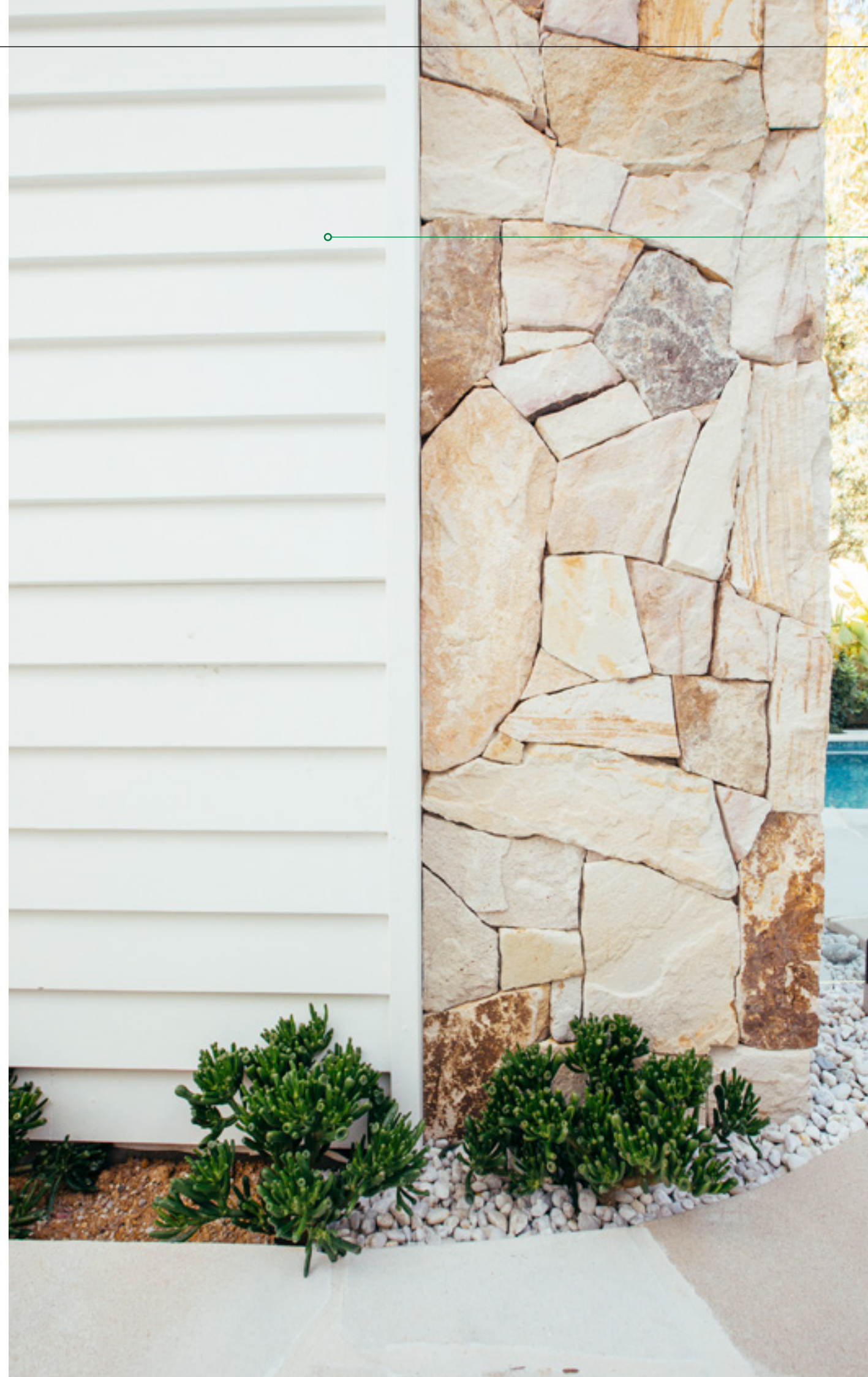
Linea™ Weatherboard 180mm
