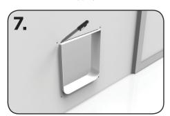
Place outer frame in hole, if the tunnel protrudes through the door, mark around tunnel.
