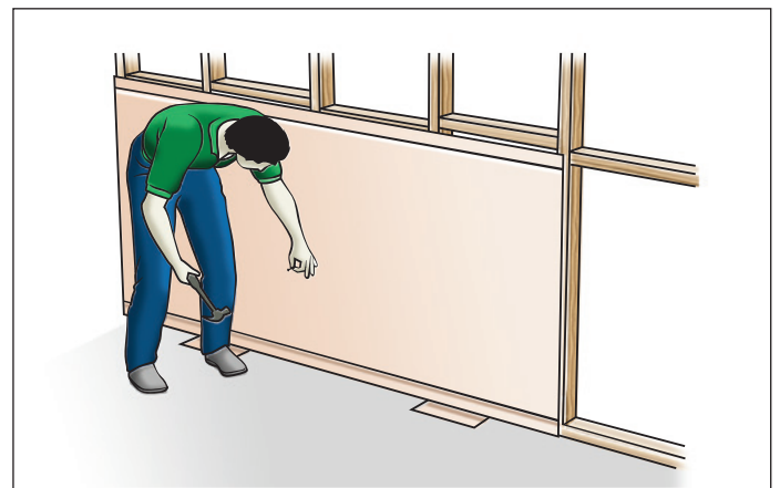
FIGURE 4 FIXING FIRST SHEET
