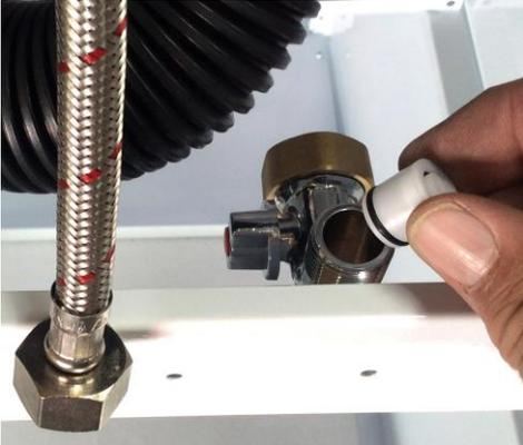
It is important to insert the valve 'O' ring end first (left photo) as the valve only allows water to pass in 1 direction. Push the valve in until it is level.
