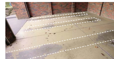
Topcoat has worn away due to tyre tracks
