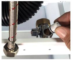
It is important to insert the valve 'O' ring end first (left photo) as the valve only allows water to pass in 1 direction. Push the valve in until it is level.
