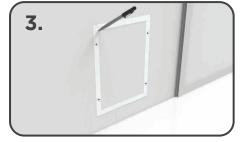
Cut out supplied template, line up height (x) with opening and trace on to door.
